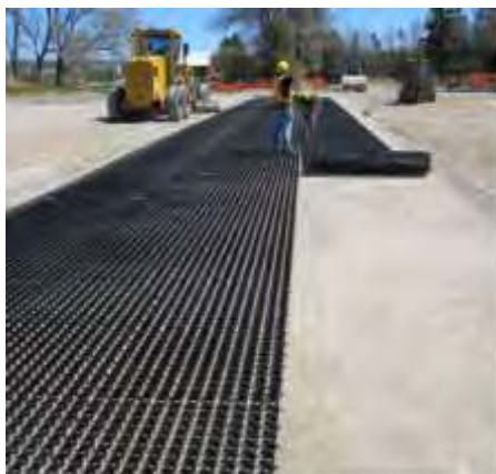
Figure 11 “Gravelpave” geocells installation
