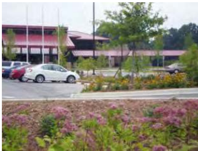
Figure 9 Linear bioretention cell in parking lot Johnston Memorial Hospital, Clayton, NC (Photo by Kim Hawkins, Hawkins Partners, Inc. in Green Infrastructure Digest 11/01/2010)
