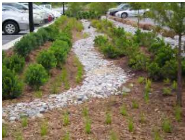
Figure 9 Linear bioretention cell in parking lot Johnston Memorial Hospital, Clayton, NC (Photo by Kim Hawkins, Hawkins Partners, Inc. in Green Infrastructure Digest 11/01/2010)
