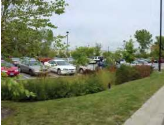
Figure 10 Bioretention area in parking lot (Photo:NRCS http://www.ia.nrcs.usda.gov/features/urbanphotos.html )
