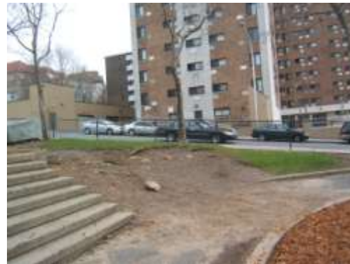
Figure 4 Eroded slope in south playground
